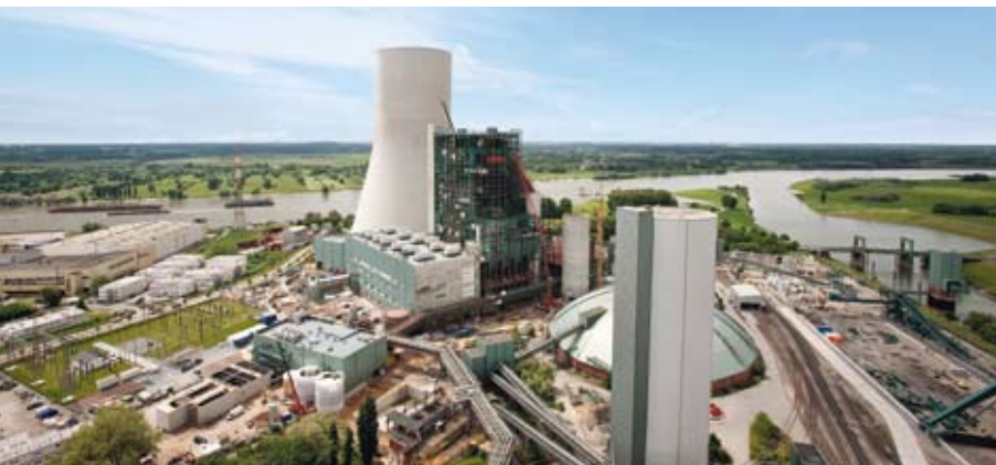
Construction in progress: the Duisburg-Walsum power plant in May 2009
