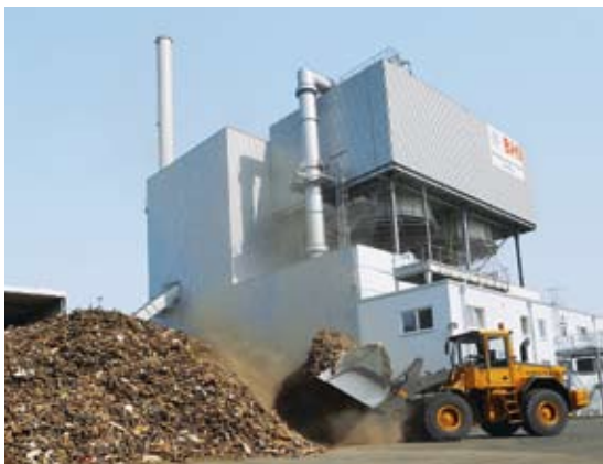
The biomass power plant in Ilmenau
