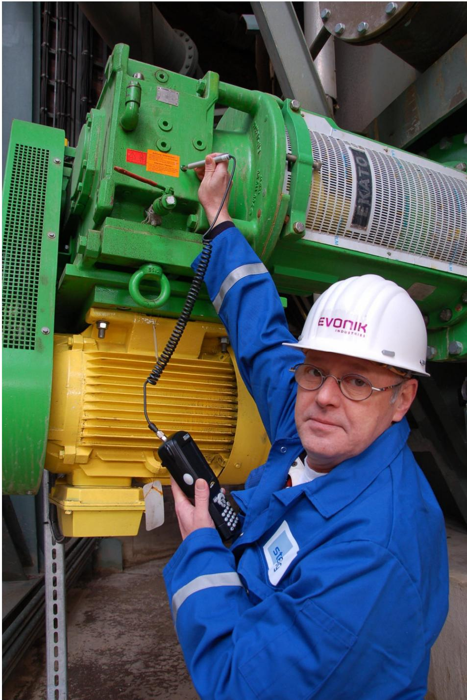
Usage of RFID-chips for maintenance
